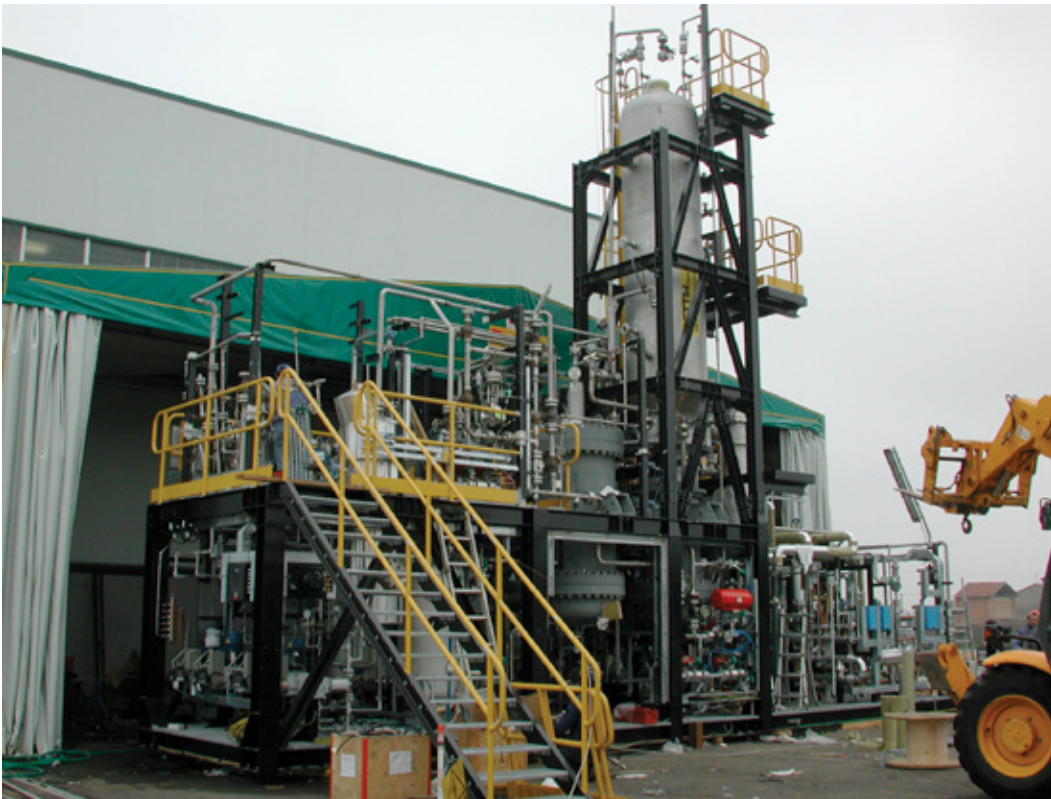
Figure 4 – Preassembly of the skids at Fores site (Forlì)
